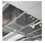
Suspension rods eliminate need for support brackets
